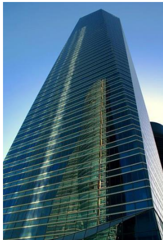
Large glass surface in new buildings
